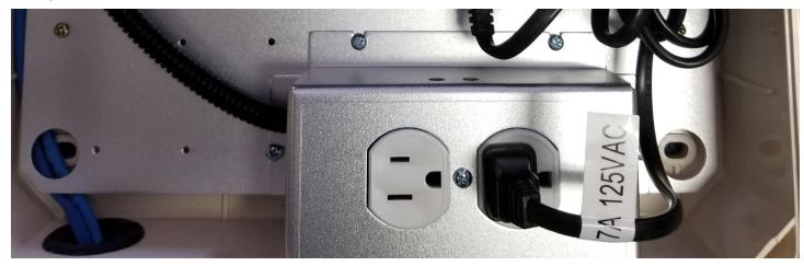
9. Connect the ventilation fan to the power card that is prewired within the enclosure.
